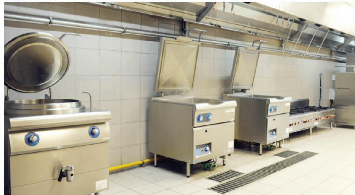
Figure 4 Example of a Central Production Unit (CPU)
